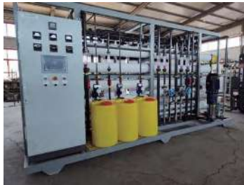
15 t/h Plant for Circulating Cooling Water
